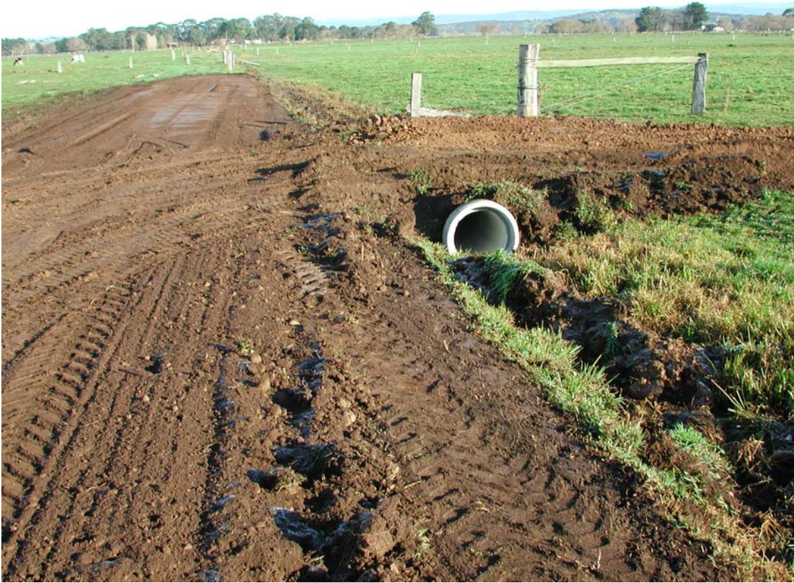
A farm track under construction. Adequate allowance has been made for drainage and the base material is being crowned and compacted using a vibrating roller
