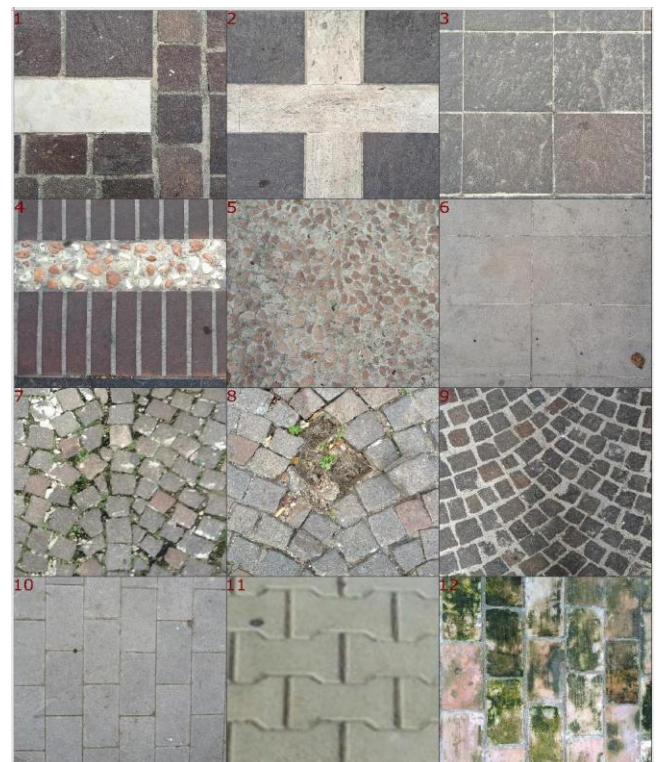
Fig. 5 The flooring types in Colonnella (limestone, porphyry stone, ...).
