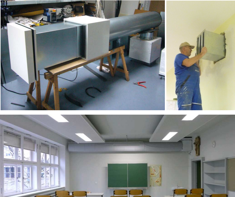
Fig. 4: Silencer and fan-box prototype manufactured by ATREA (top-left), mounting of silencer in the wall (top-right), fan box and textile diffuser in operation (bottom)
