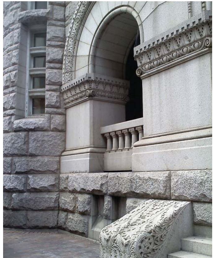
Fig. 3. Stone walls with substantial mass have high thermal inertia.
