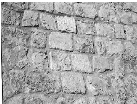
Fig. 9. Fortification masonry facing the National Stadium of Heraklion in Crete.
