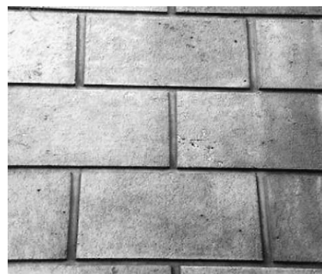
Fig. 2. Kapandriti's stone surface at the Bank of Greece historic building in Athens.
