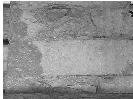
Fig. 10. Western facade of the Tobacco Cutting Factory in Heraklion, Crete.
